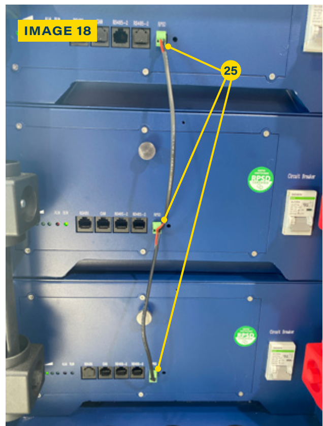
25 RAPID SHUTDOWN DAISY CHAINING
