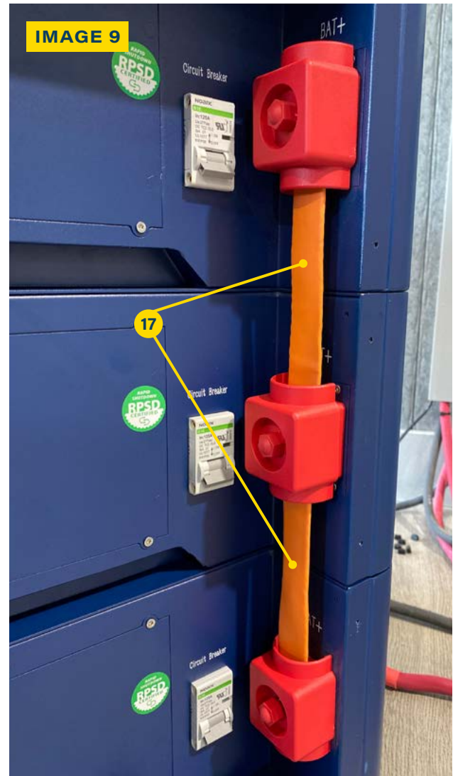
17 PARALLEL BATTERY CABLE
