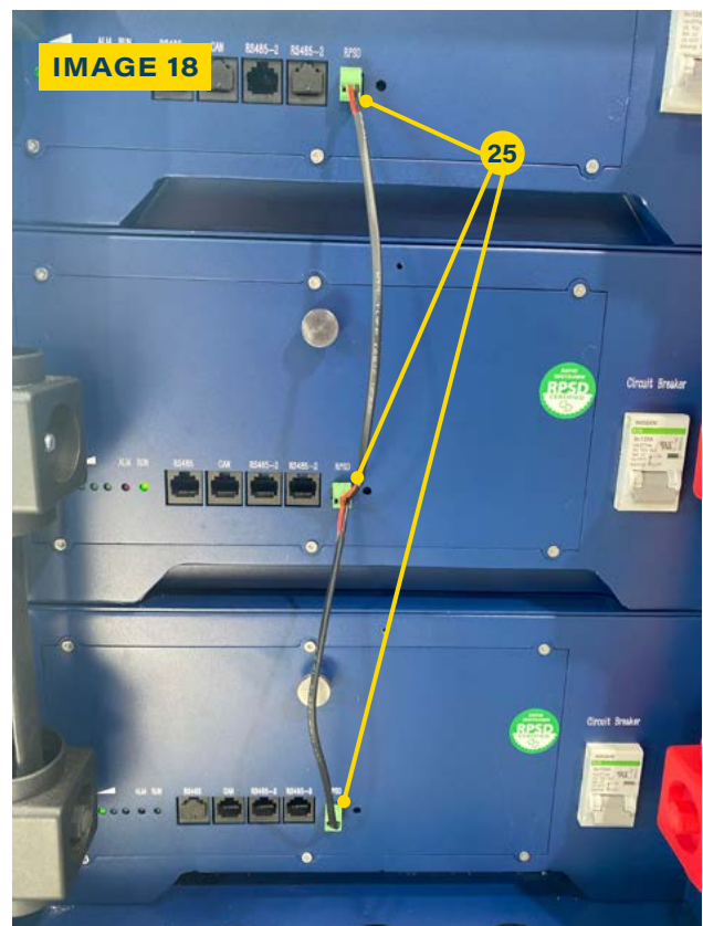
25 RAPID SHUTDOWN DAISY CHAINING
