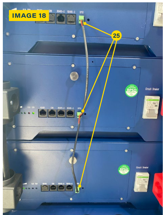
25 RAPID SHUTDOWN DAISY CHAINING
