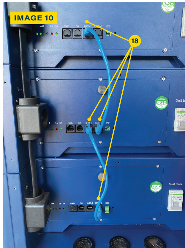
18 USE INCLUDED NETWORK CABLES TO DAISY CHAIN BATTERIES FROM RS485-2 PORTS.
